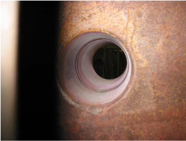
Nozzle welds were RT and LPI tested.
