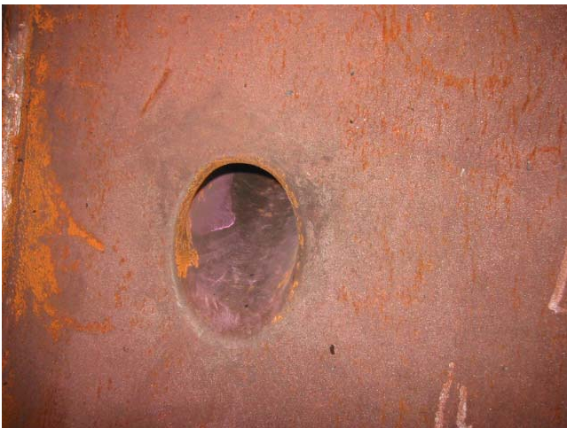
Penetrations were acceptably profiled.
