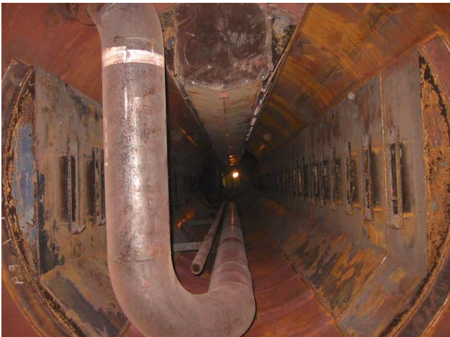
Internals being completed.
